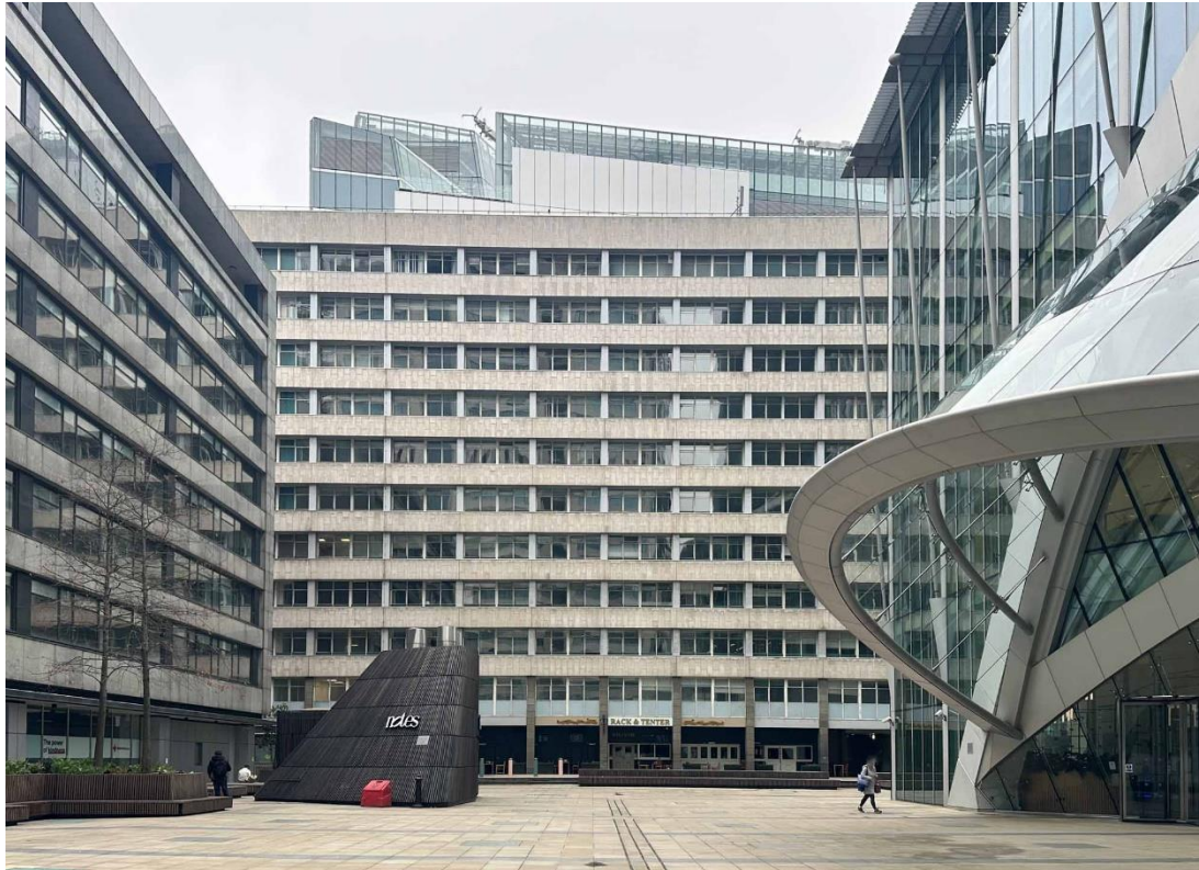
Image 1: North elevation of original building from City Point Plaza
