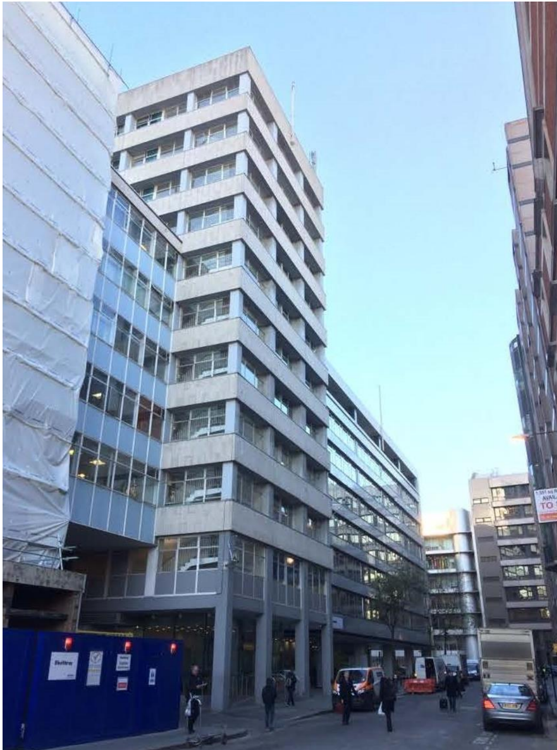
Image 5: East elevation of original building from Moorfields
